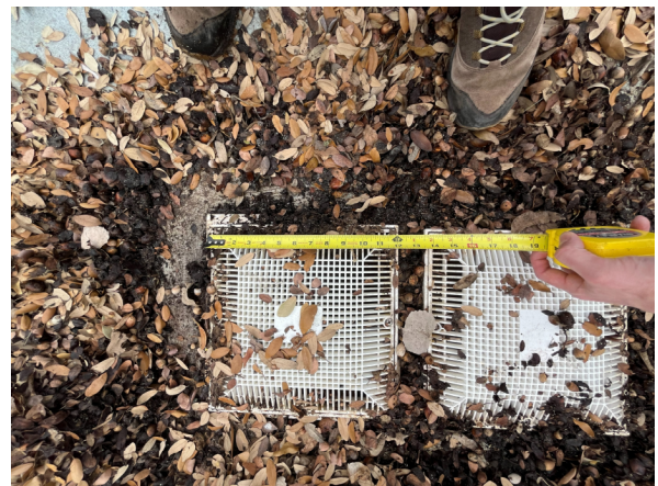
Photo #30 View of the 12" x 12" domed main drains (four (4) instances).
