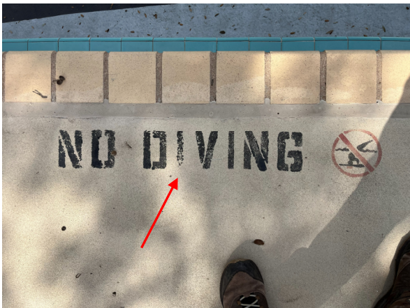
Photo #3 Example view of warning signage on the Lap Pool deck.
