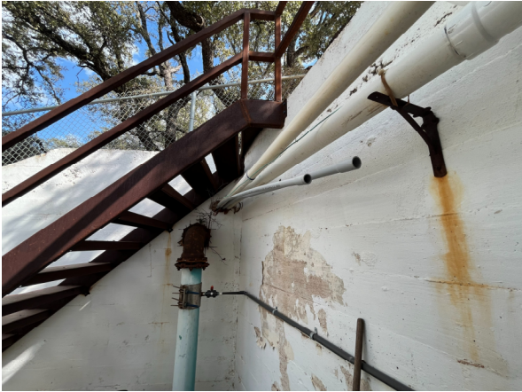
Photo #42 View of Lap Pool return piping.
