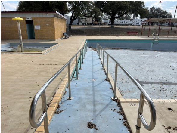
Photo #13 View of the ramp entry and handrails leading into the Lap Pool.
