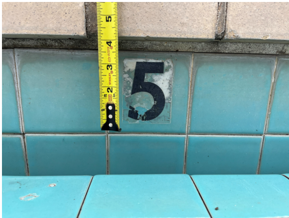
Photo #27 Example view of 3" tall vertical depth marking on the Lap Pool walls.
