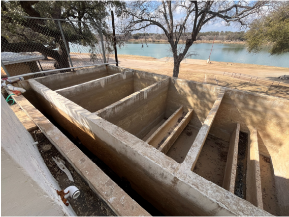
Photo #35 View of existing Lap Pool vacuum sand filter pits.
