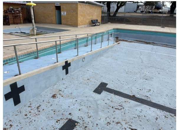
Photo #10 Example view of the Lap Pool lane markers and wall targets.
